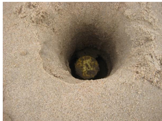
Figure 1: Installation of a drainage tube below the beach surface
