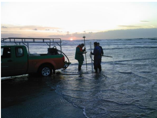
Figure 1: Installation of a drainage tube below the beach surface
