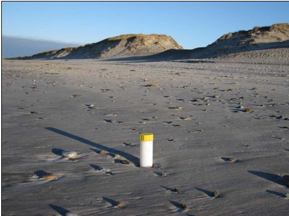
Figure 5-24 Exposed vertical drainage tube after a storm near Hvide Sande, Denmark
